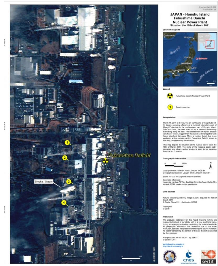
Japan, Honshu Island, Fukushima Daiichi Nuclear Power Plant, situation the 16th of March 2011, Credits : SERTIT
