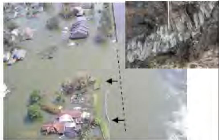
**Displacement of wall and part of levee**
